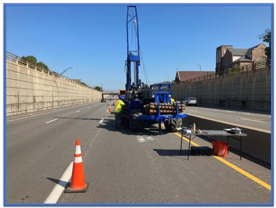
Photo 2 – CME setting up the drill rig within the left lane of the westbound traffic (with WZTC) along Route 33, Kensington Expressway for the geotechnical and environmental investigation.
